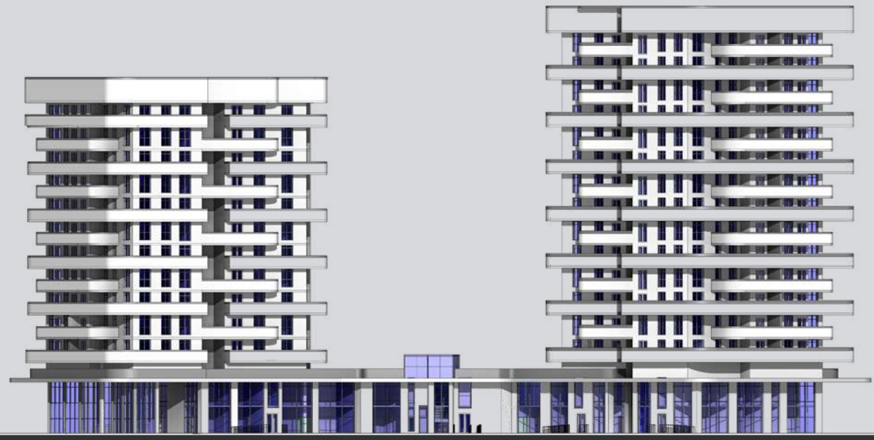
Facade from the entrance to the residential cells
